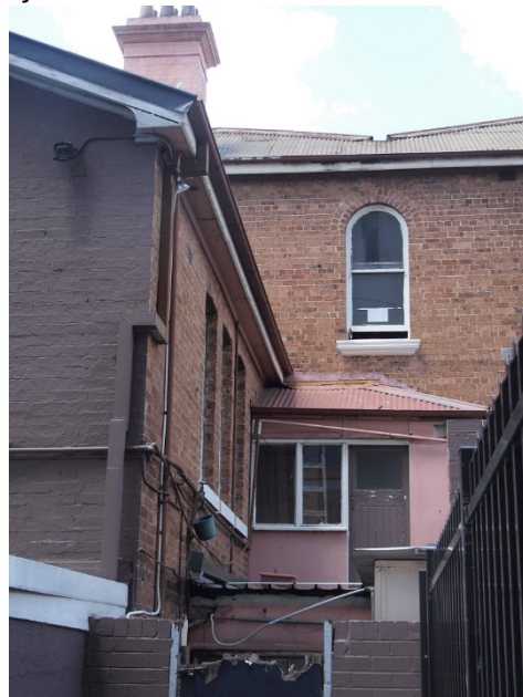
Figure 4 Space FF16 (pink colour) that could form the model of a two level verandah on this elevation to reduce impacts from the loss of overall form if the Northern wing was approved for removal.
